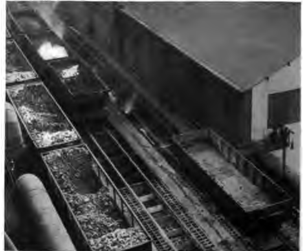
Fig. 4. Grill-Work Protection over Ore, Coke, and Limestone Bins at Blast Furnaces.*
